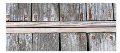
A loose edge bumper (right) on an inner basin float may eventually fall in the water, causing pollution and losing protection for any docked boats.
