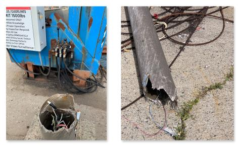
Crane operator could stumble and fall backwards onto jagged fiberglass light pole base. Also, exposed electrical wiring presents an electrocution hazard. Anyone could have impaled an ankle on the jagged end of the pole. This condition has existed from around 2022 March 27. The fallen pole was removed four months later.
