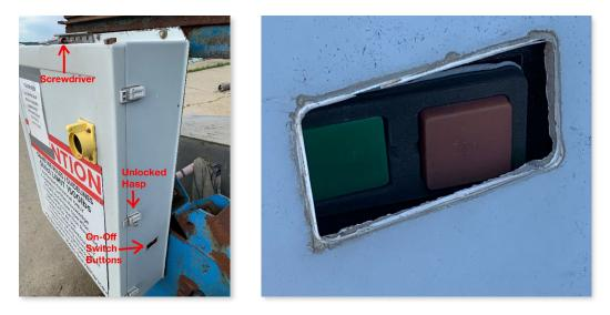
Keyswitch was being switched on and off with a screwdriver (seen atop the box) since 2021. On-off switchbuttons on the bottom right side of the box (closeup view is photo on the right) were loose, pushed inside the box, allowing rain and salt spray to enter the box. This box was replaced on August 1 or 2 after the issue was escalated.
