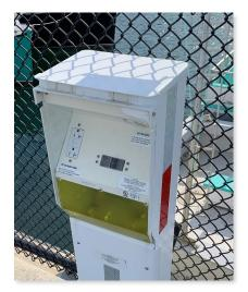
This is **one of six (6) outlet boxes that have lost their weather covers,** allowing water and salt spray to corrode plug connections and circuit breakers. They are still missing protection from the elements–some missing since a year after pier reconstruction.
