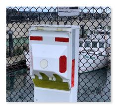
This outlet box has an intact weather cover, protecting outlets and circuit breakers from rain, ice, and salt spray. All outlet boxes should have this weather cover protection
