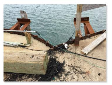
In late 2019, electric wiring at the Fish Pier base (above left) existed *outside* an enclosure. The exposed wiring and conditions (above right) were reported on 2016 April 22, and were eventually fixed.
