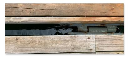
Below left shows how two segments of floating pier are properly constructed to prevent feet from getting caught in the gap between segments.
