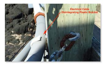
There are a great number of plastic conduit brackets on the south side of the Fish Pier. Many broken brackets remain, even while absent any conduit. The plastic disintegrates, dropping plastic into the water, adding to plastic pollution in the sea, endangering sealife.
