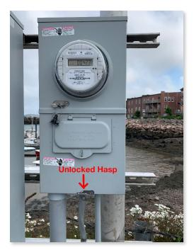
Anyone has access to the wiring inside this circuit box that has been unlocked since at least 2021.
