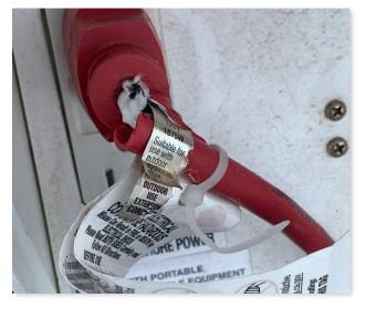
Insulation on this cable is broken down to the internal wiring. At this writing the female end of this cable is submerged along the west edge of the inner basin (see image on page 14). This condition has existed for over a month, even after informing the Eastport Port Authority director in person on 2022 July 29.
