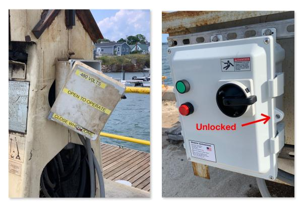
The north crane 480-volt control circuit box (above left) is in poor condition. The unlocked 480-volt south crane control circuit box (above right) is the same kind that has just replaced the 480-volt box on the Fish Pier crane (shown on pages 4 & 5).
