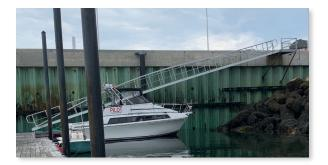
The inner basin ramp (above left and top) is considerably shorter than the north floating piers ramp (above bottom right), making the inner basin ramp very steep at low water, and dangerously slippery when wet from rain. Winter conditions make it even more hazardous. **Suggestion:** Extending the inner basin ramp would make using the ramp much safer.
